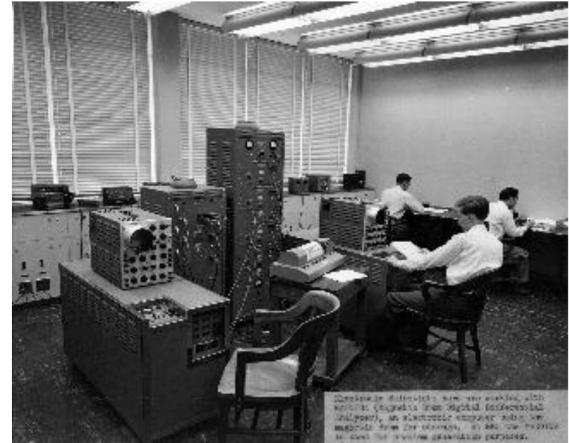
MADDIDA (Magnetic Drum Digital Differential Analyzer, Northrop Aircraft) 1952
